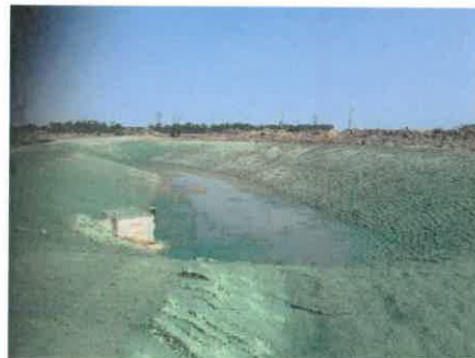
Figure 4- Temporary or permanent seeding applied to all denuded areas during all phases of construction
