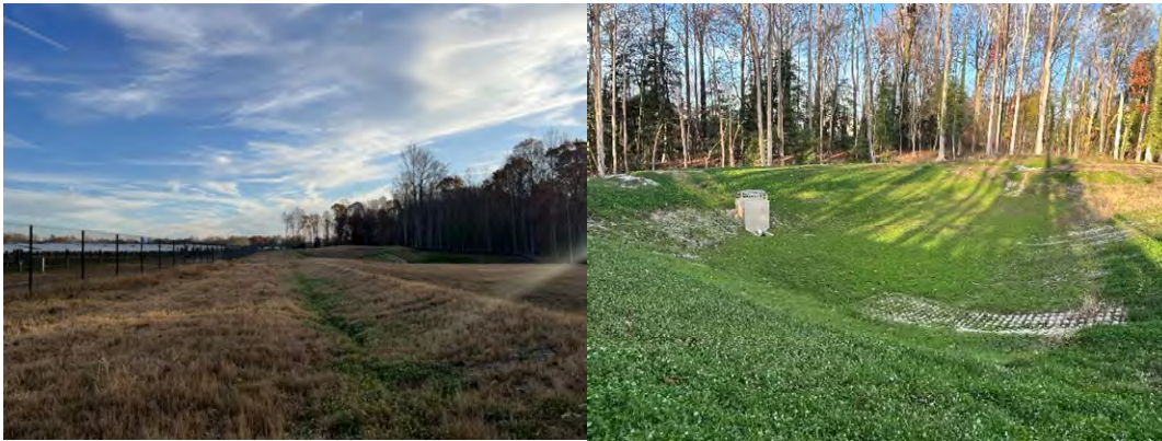
Figure 3– Diversion Channels and Stormwater Management Ponds
